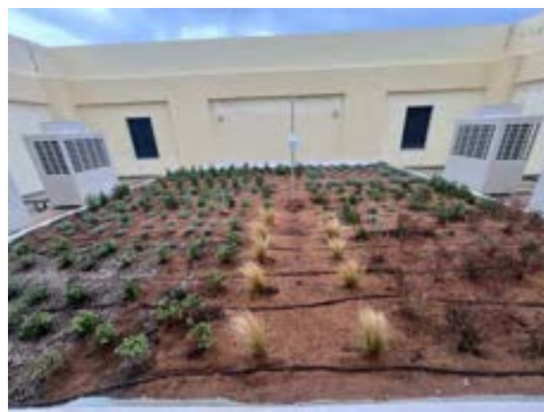
Figure 2: Completed green roof at TUC
